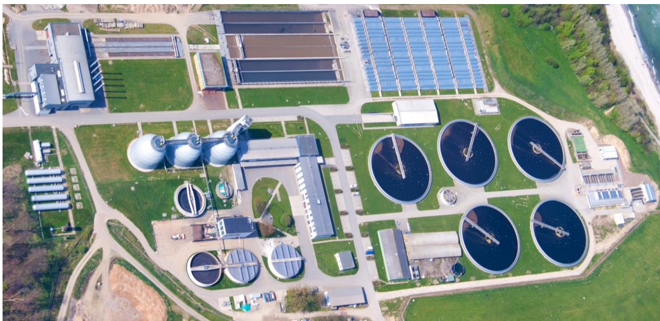
Purification Plant (© Louis-F. Stahl / WikiCommons. CC BY-SA 3.0; Link ).
